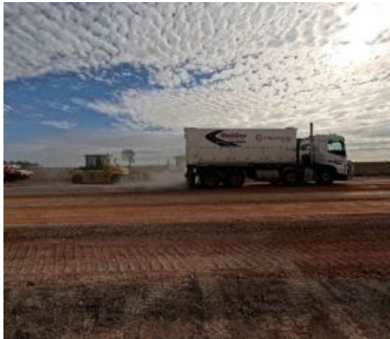
Figure 8 — Floraville Road: Zone 2 cement stabilisation, June 2026
