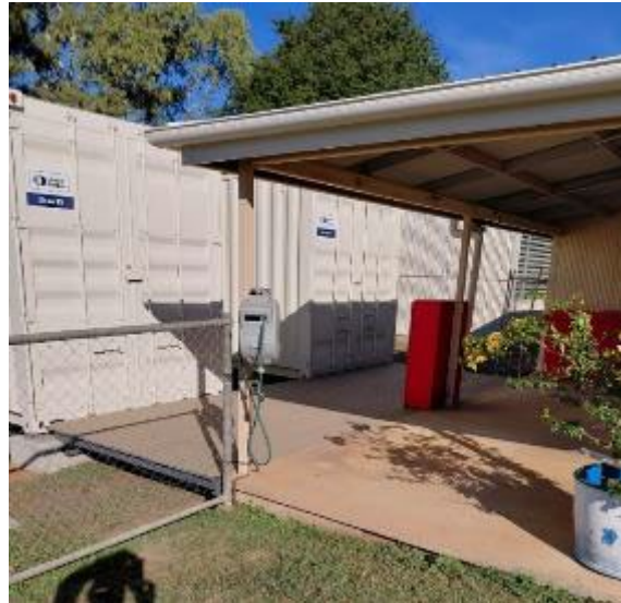
Figure 1: The two archive containers connected to the Admin Building.
