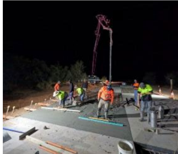
Figure 7 — Floraville Road: Stage 4 concrete floodway pour, May 2026
