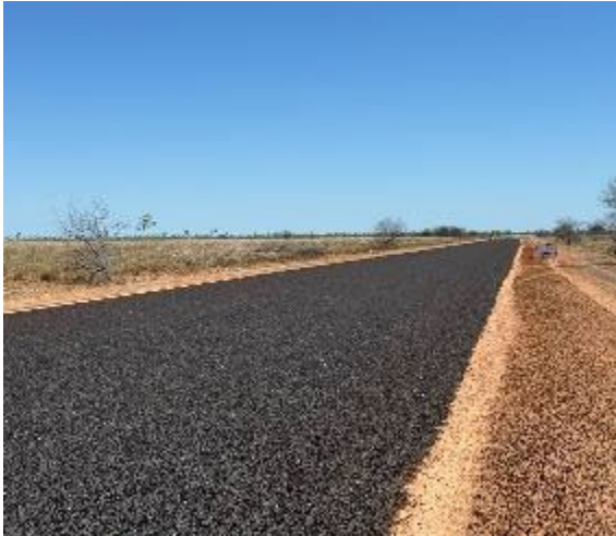
Figure 6 — Floraville Road: Zone 1 pavement spray seal complete, June 2026
