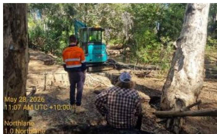
Figure 10 - Test-pitting at Lawn Hill Creek Crossing under Waanyi supervision, May 2026
