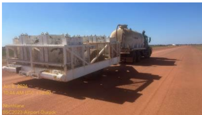
Figure 1 —Base course proof rolling (MARCO roller) on the interim runway, June 2026
