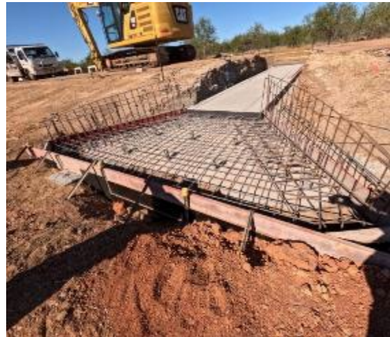
Figure 9 — Floraville Road: Culvert 4 headwall and apron reinforcement, June 2026
