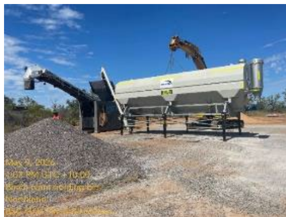
Figure 5 — Concrete batch plant established, May 2026
