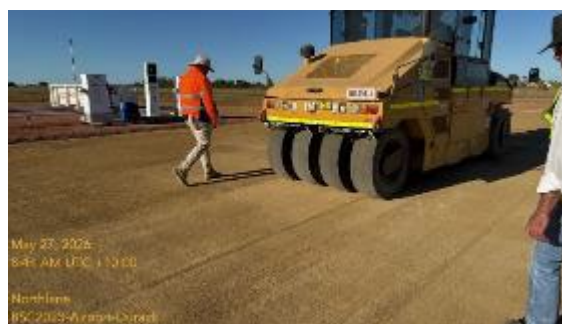
Figure 3 — Temporary Apron following passing proof roll, May 2026
