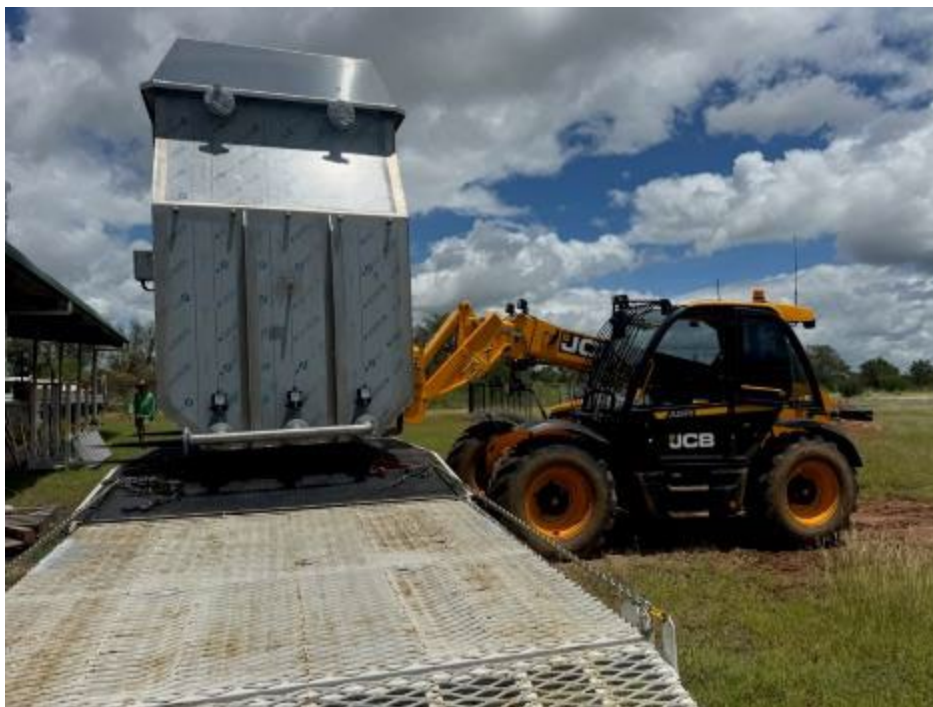
Figure 3: The Clarifier unit being installed at the GWTP.
