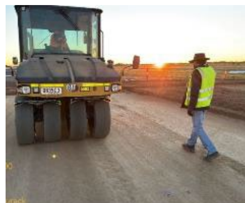
Figure 12 — Burketown Airport: Proof-roll inspection on the interim runway, June 2026
