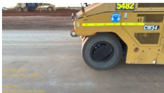
Figure 2 —Cement stabilisation remediation of the Main Runway southern node, May 2026
