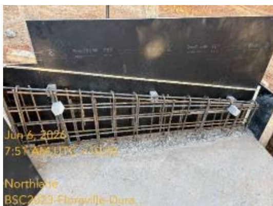
Figure 11 — Floraville Road: Pre-pour QA inspection, June 2026
