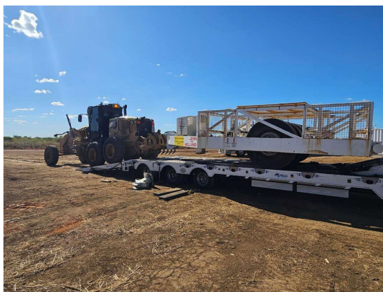
Figure 2 — Specialised plant (MARCO Roller) arriving, May 2026
