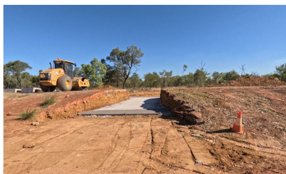
Figure 9 — Floraville Road: Culvert Construction (12 May 2026)
