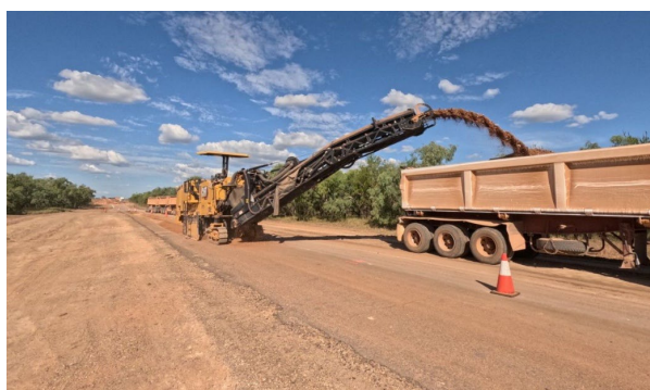
Figure 8 — Floraville Road: Zone 1 Road Excavation (5 May 2026)
