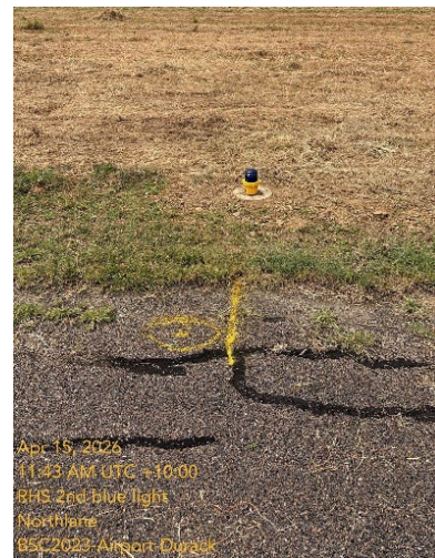
Figure 12 — Airport: Lighting QA Inspection
