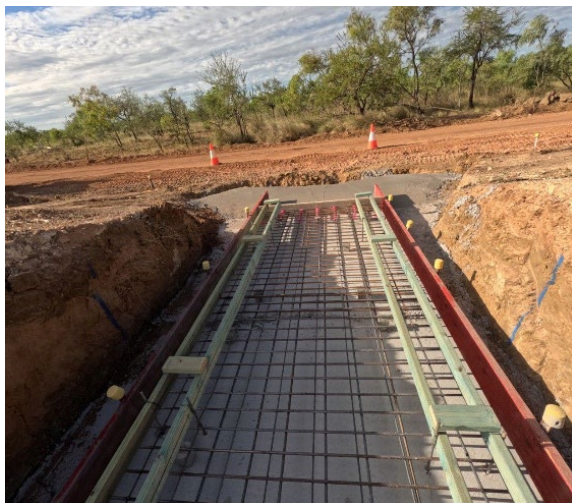
Figure 11 — Floraville Road: Pre-Pour QA Inspection
