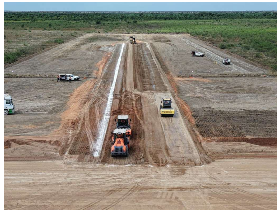
Figure 1 — Padfoot rollers compacting the second pass of lime stabilisation, May 2026
