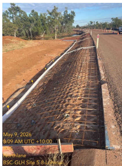
Figure 5 — GLH Site 5: Mesh Installation, RHS, 9 May 2026
