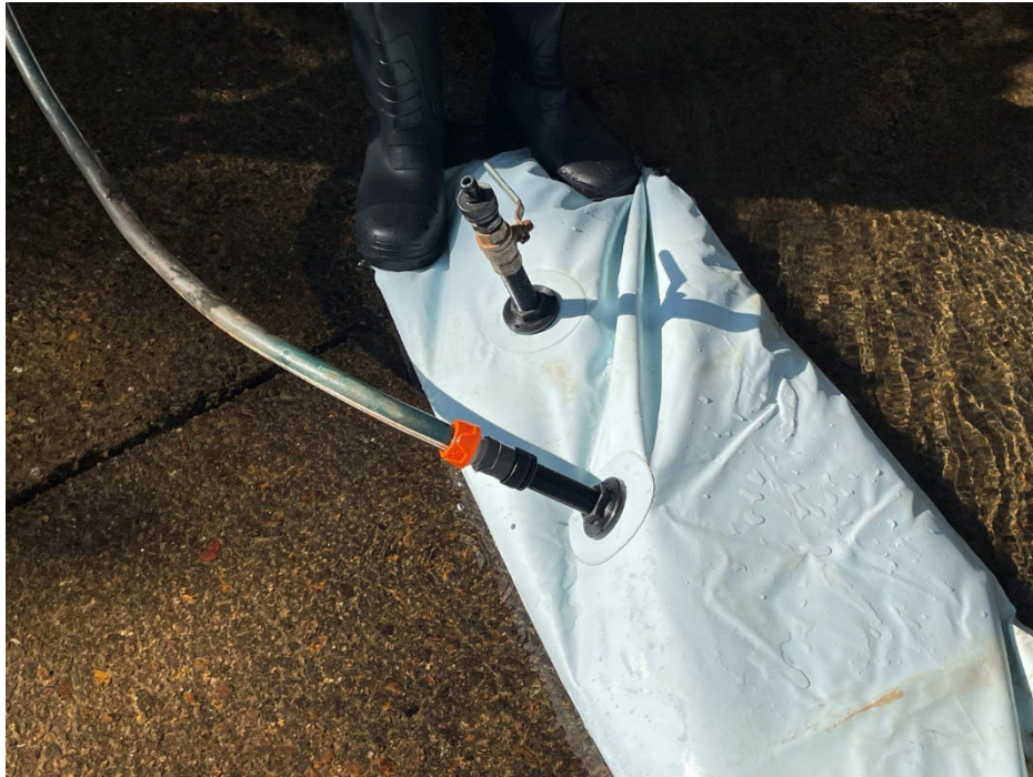
Refilling the water barrier tube
