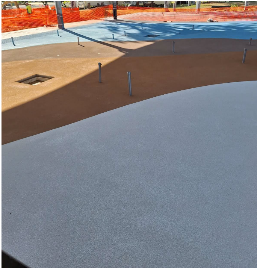
Figure 1: Slab of the Splash Park (wet area) poured and painted
