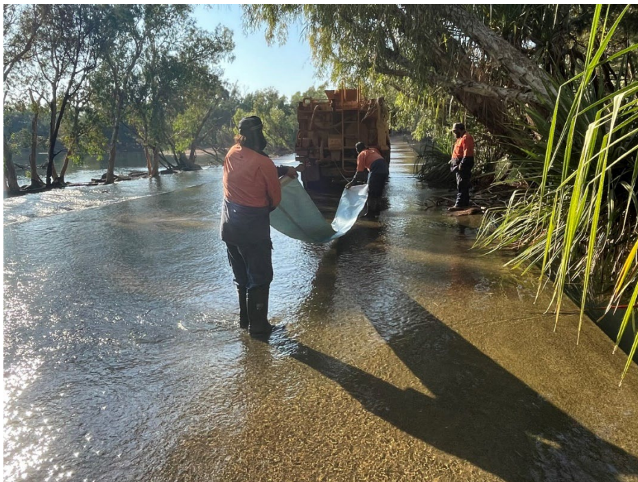
Road crew unrolling the 20m water barrier tube
