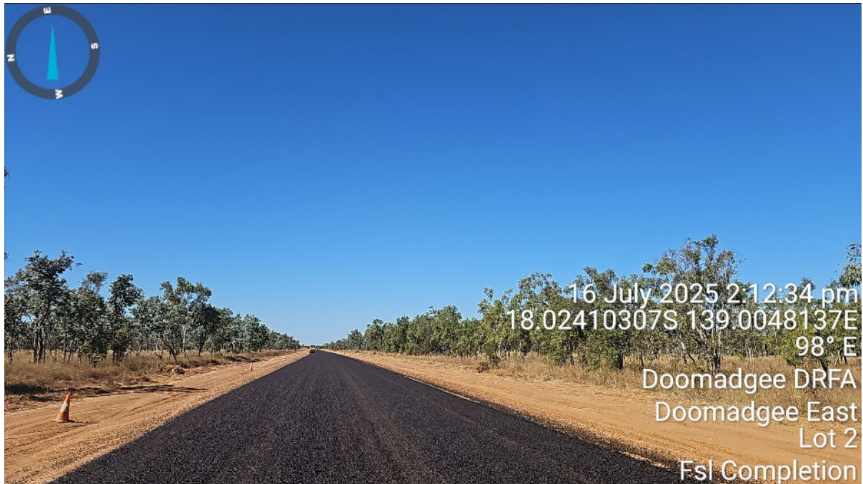
Doomadgee East Road – Seal installed
