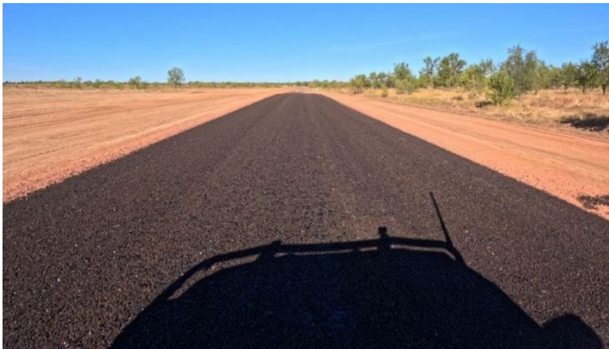
Truganini Road – Patch Repair, Seal installed
