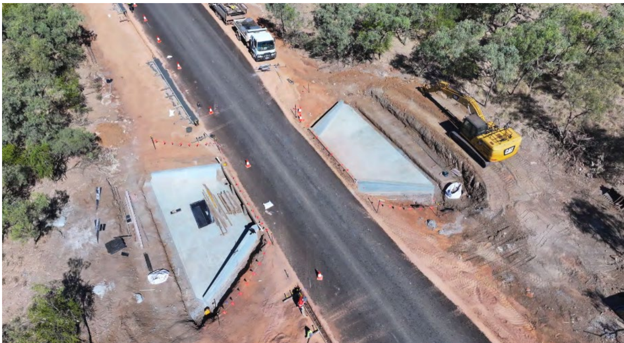
Floraville Road – Seal installed, Concrete Works
