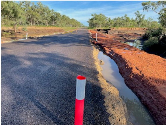
Photo 9: Jack's Gully flood damages
