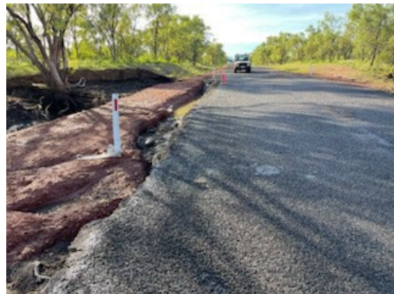
Photo 8: Jack's Gully flood damages
