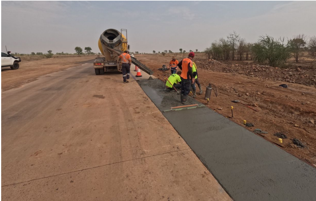
Image 5 – Floraville Road – Floodway Widening Works
