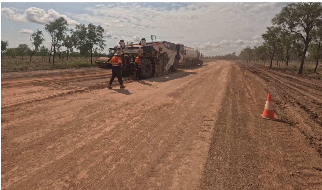
Image 6 – Floraville Road – Stabilising Works
