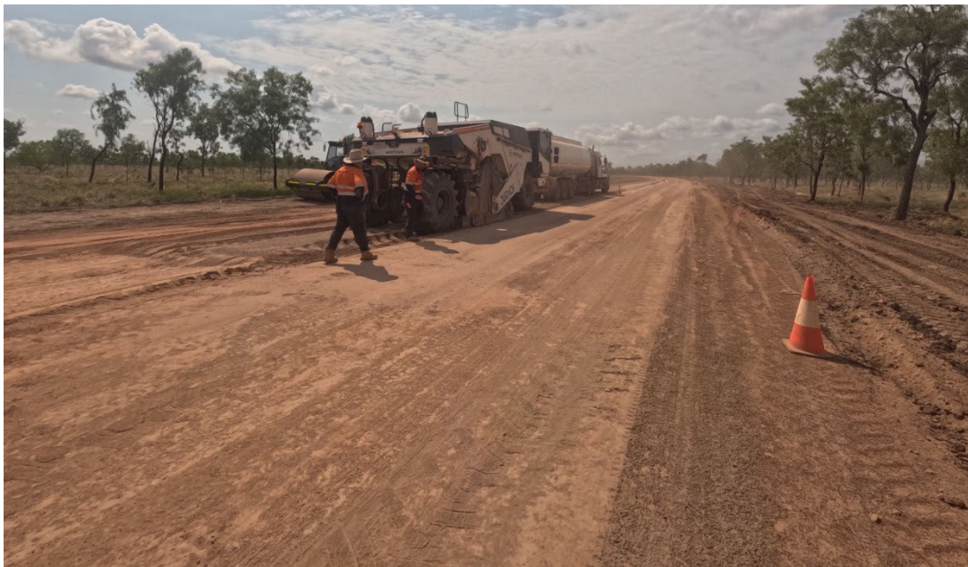
Image 6 – Floraville Road – Stabilising Works
