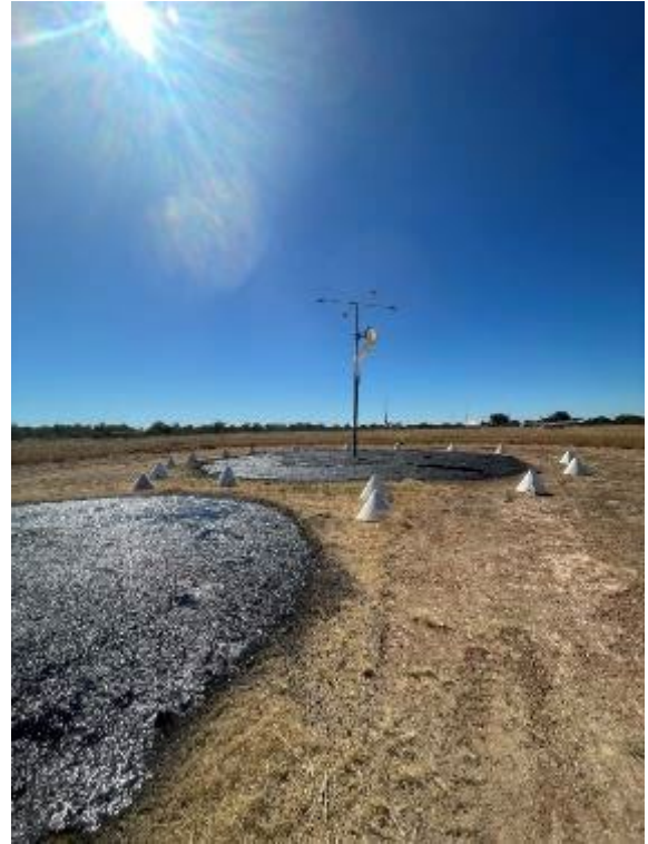
Airport windsock and signal circle bitumen spraying
