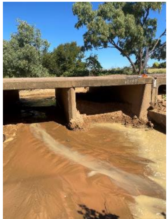
Flushing silt
