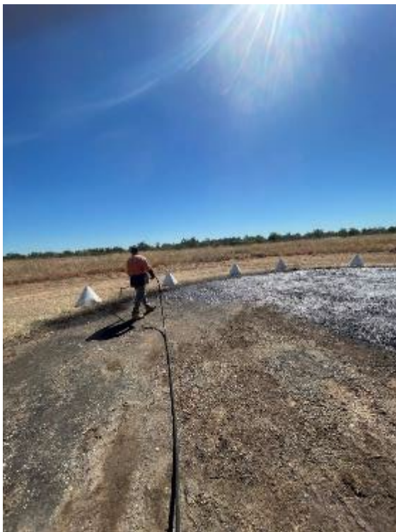
Bitumen spraying wind sock circle area
