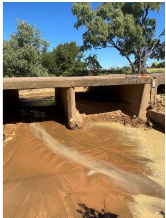
Flushing silt
