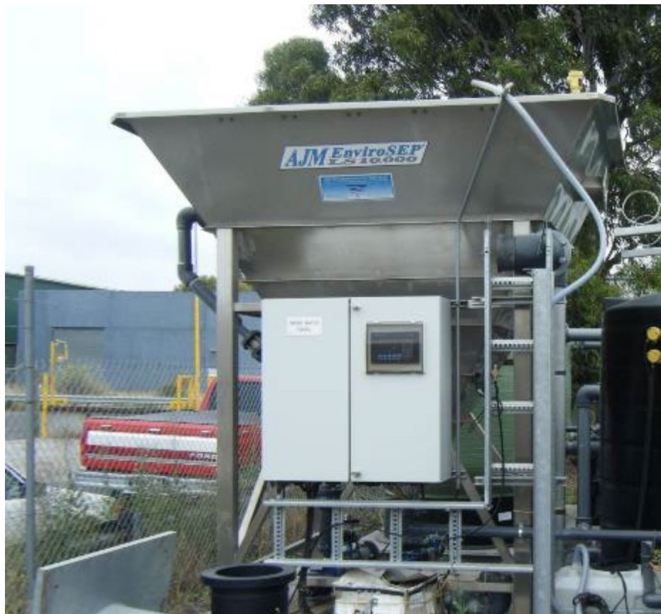
Figure 2: Lamella clarifier located at Richmond.
