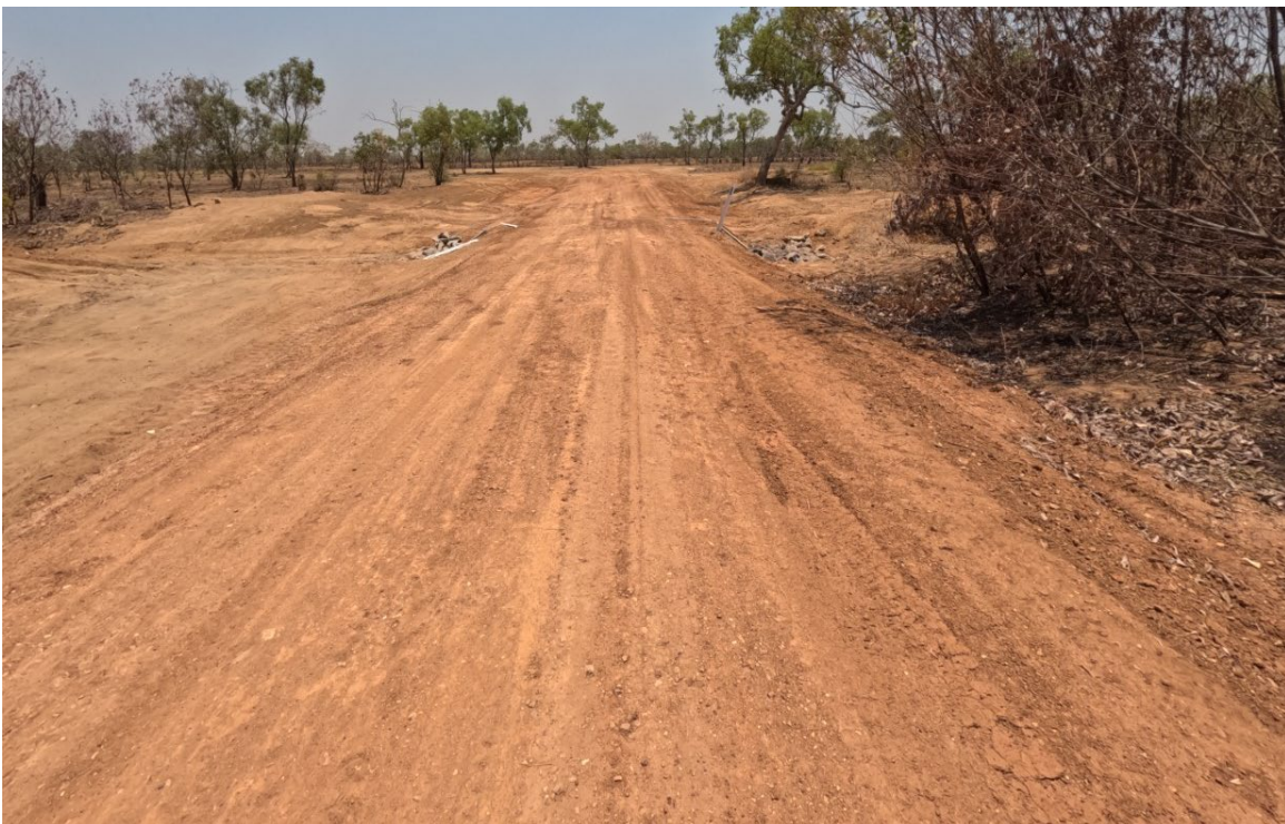
Figure 4: Bowthorn Rd Culvert Replacement
