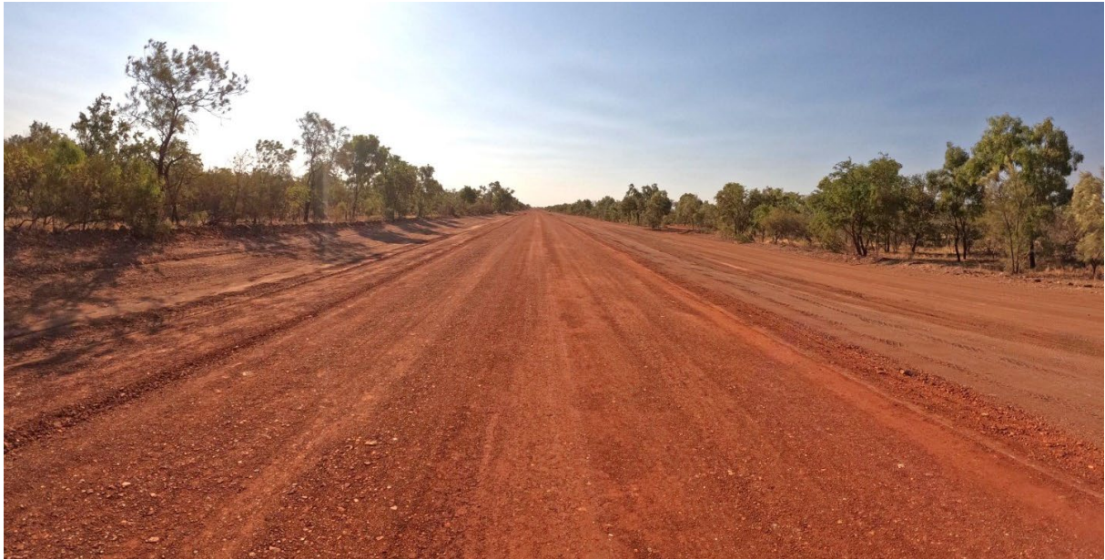
Figure 1: DRFA (Restoration) works are in progress along Gregory Lawn Hill Road
