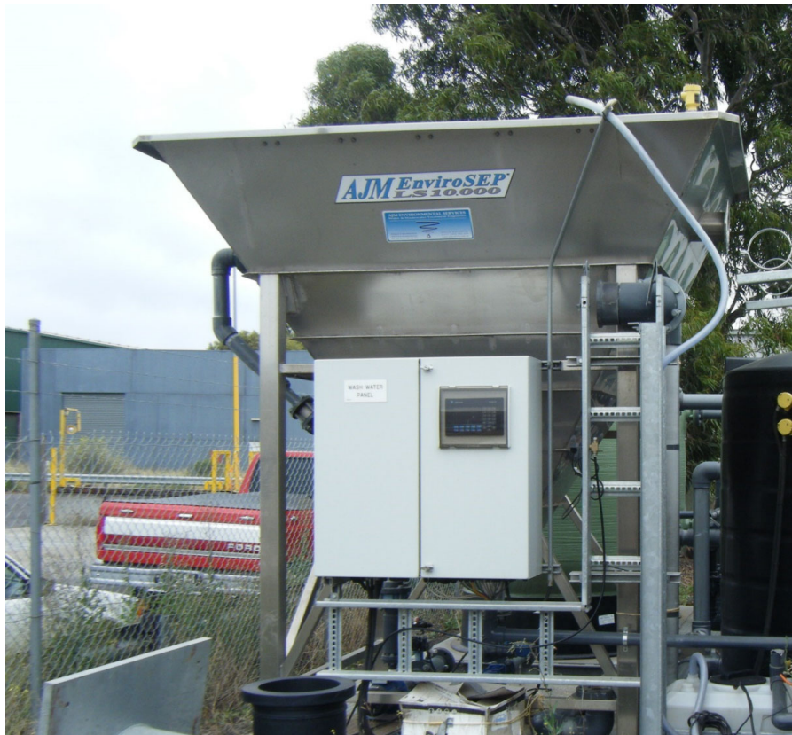
Figure 1: Lamella clarifier located at Richmond
