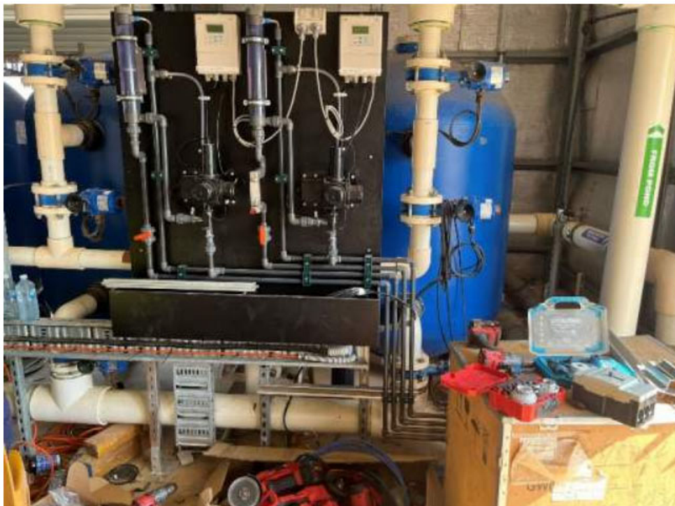
Figure 1: Installation of BWTP Water Quality Analyser and the hardware
