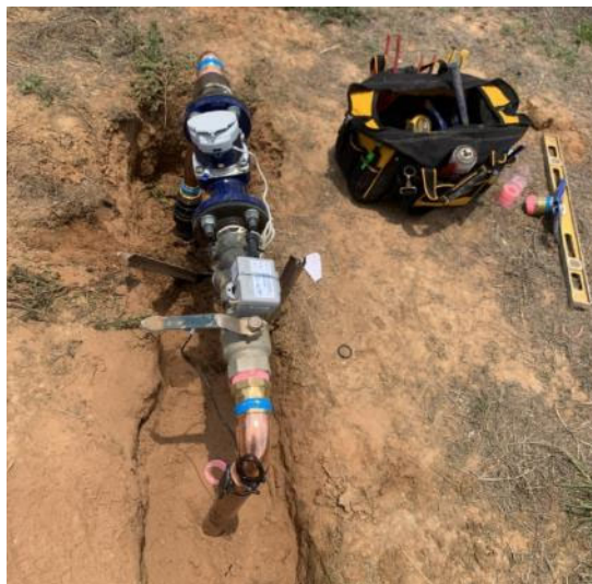
Figure 5: Installation of a DN50 Smart Water Meter
