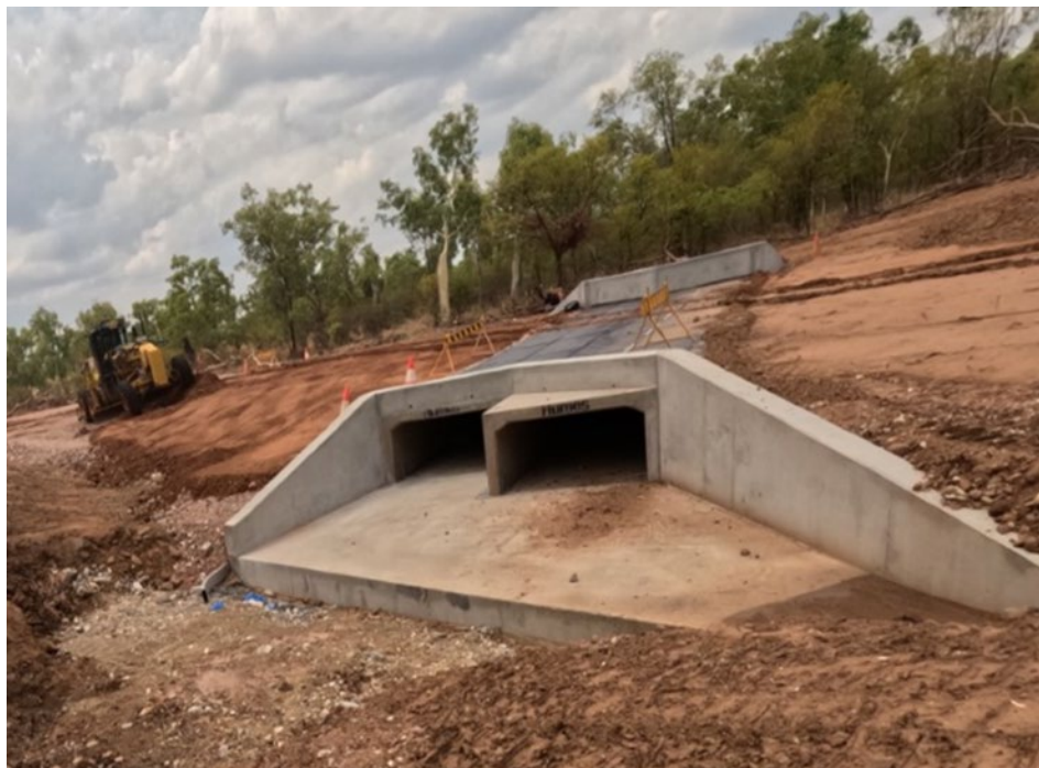
Figure 4: Dinner Creek Culvert – completed wingwalls
