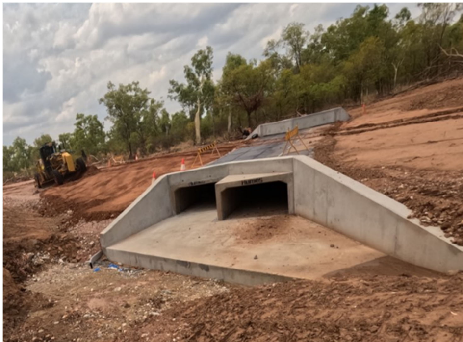
Figure 4: Dinner Creek Culvert – completed wingwalls
