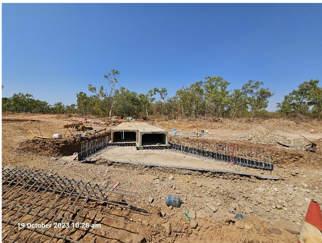
Figure 4: Dinner Creek Culvert – before the concreting of wingwalls
