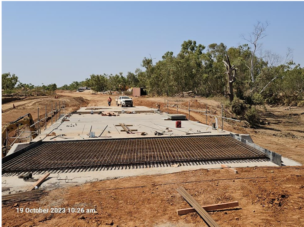
Figure 3: Archie Creek Culvert – before completing the approach slab
