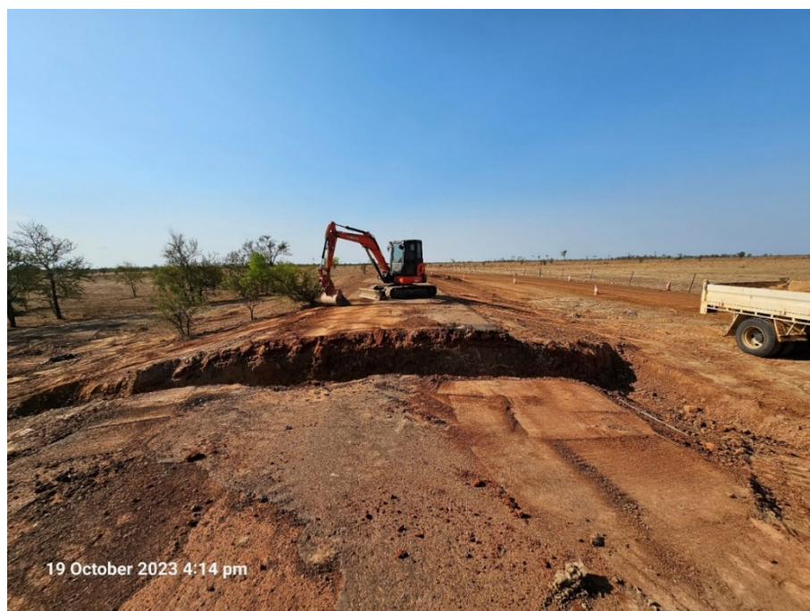
Figure 6: Site 12 Culvert – completed excavation works.
