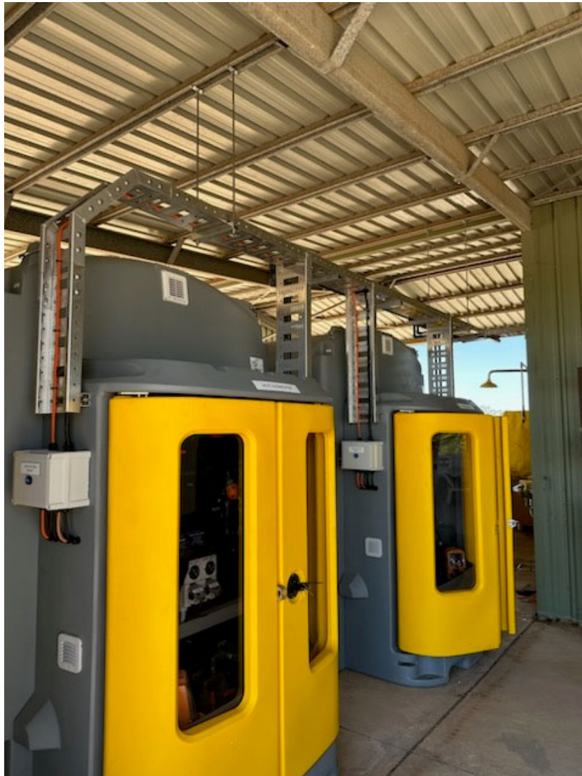
Figure 1: New Chemical dosing pods at Gregory Water Treatment Plant
