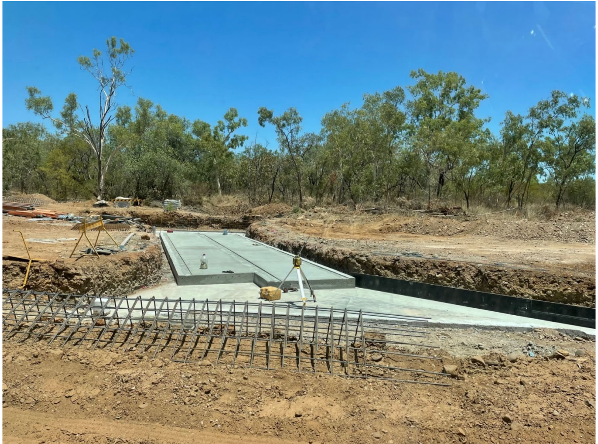
Figure 4: Dinner Creek Culvert Base
