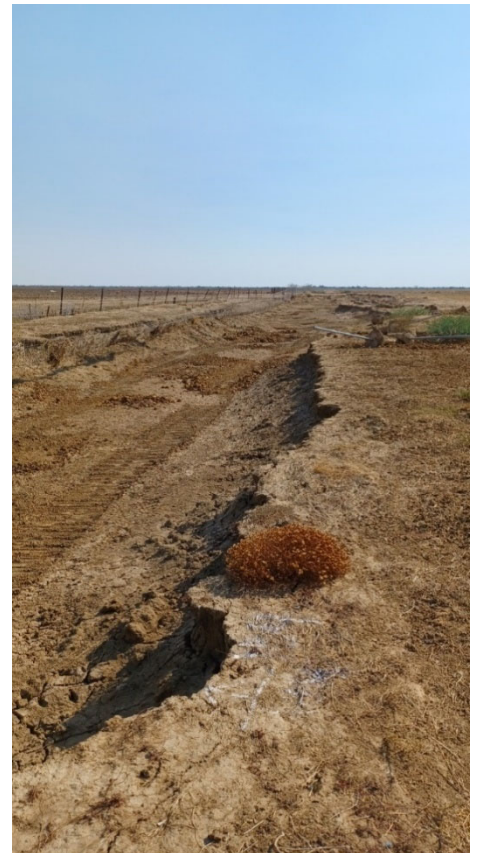
Figure 11 - Scour on east side of Burketown runway
