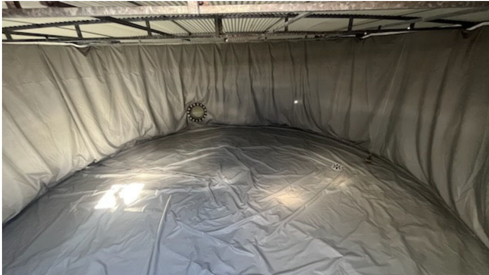
Figure 9. After liner installed
