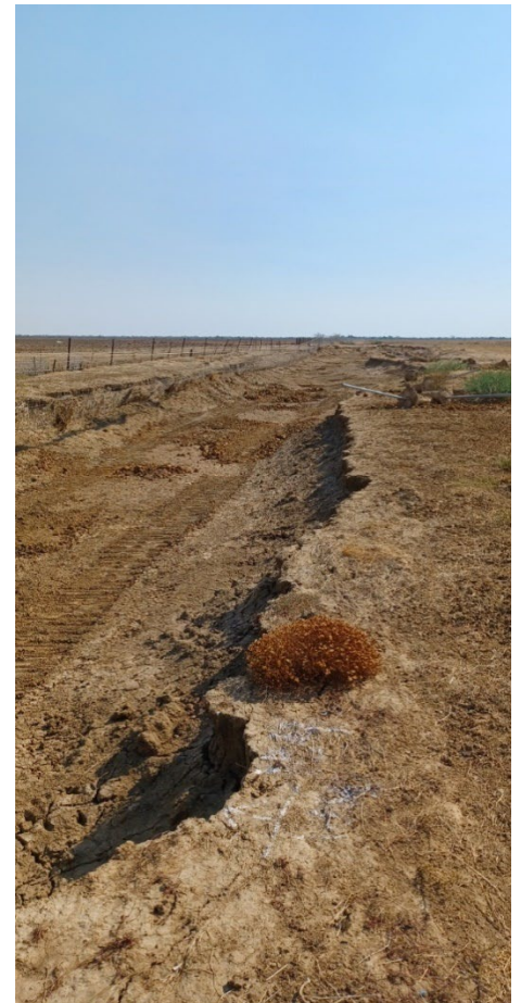
Figure 11 - Scour on east side of Burketown runway
