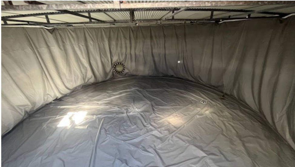
Figure 9. After liner installed
