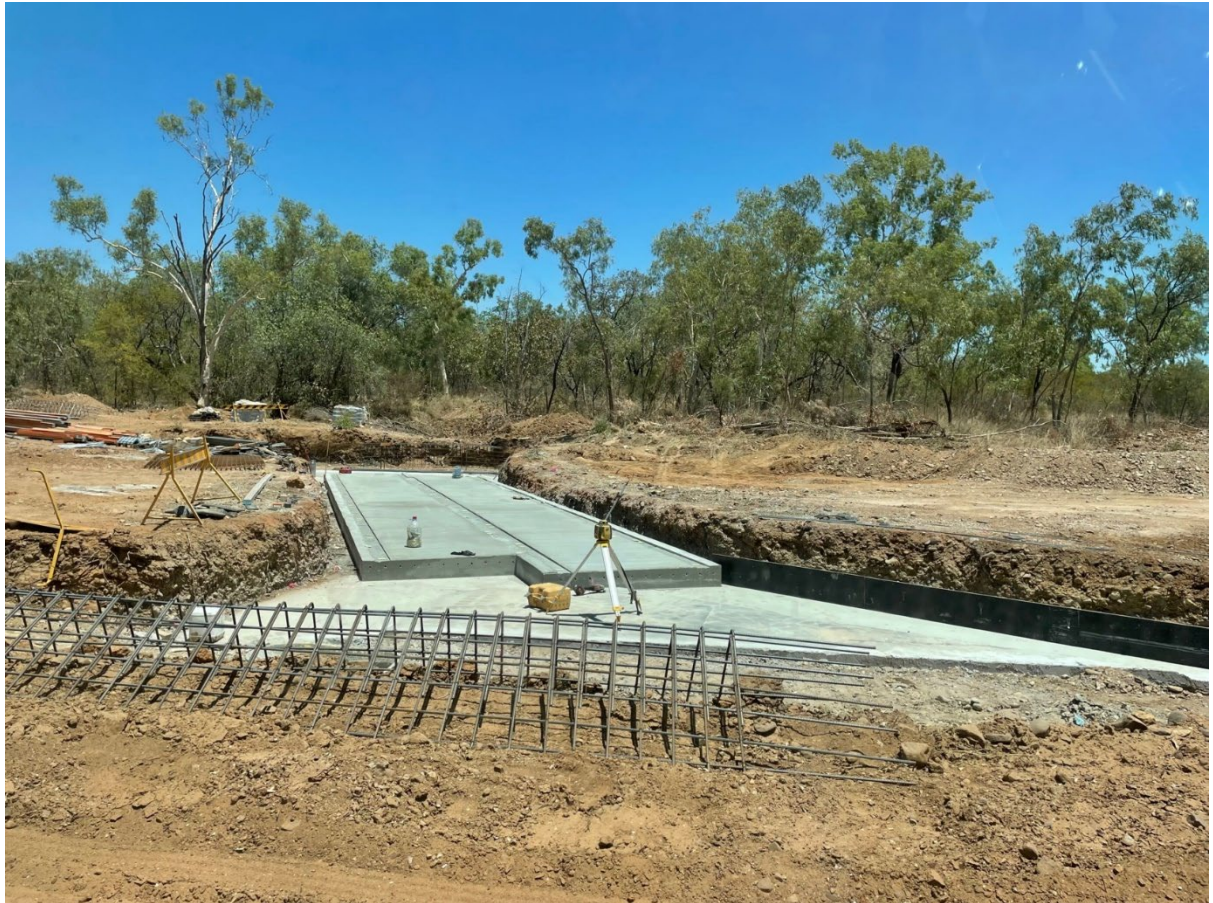
Figure 4: Dinner Creek Culvert Base
