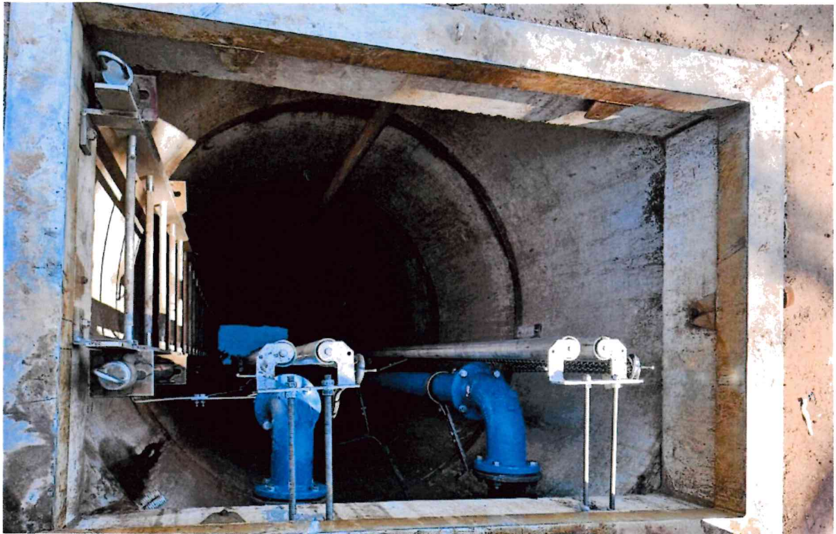
Figure 1: Gregory Raw Pump well including new suction pipe and pump
