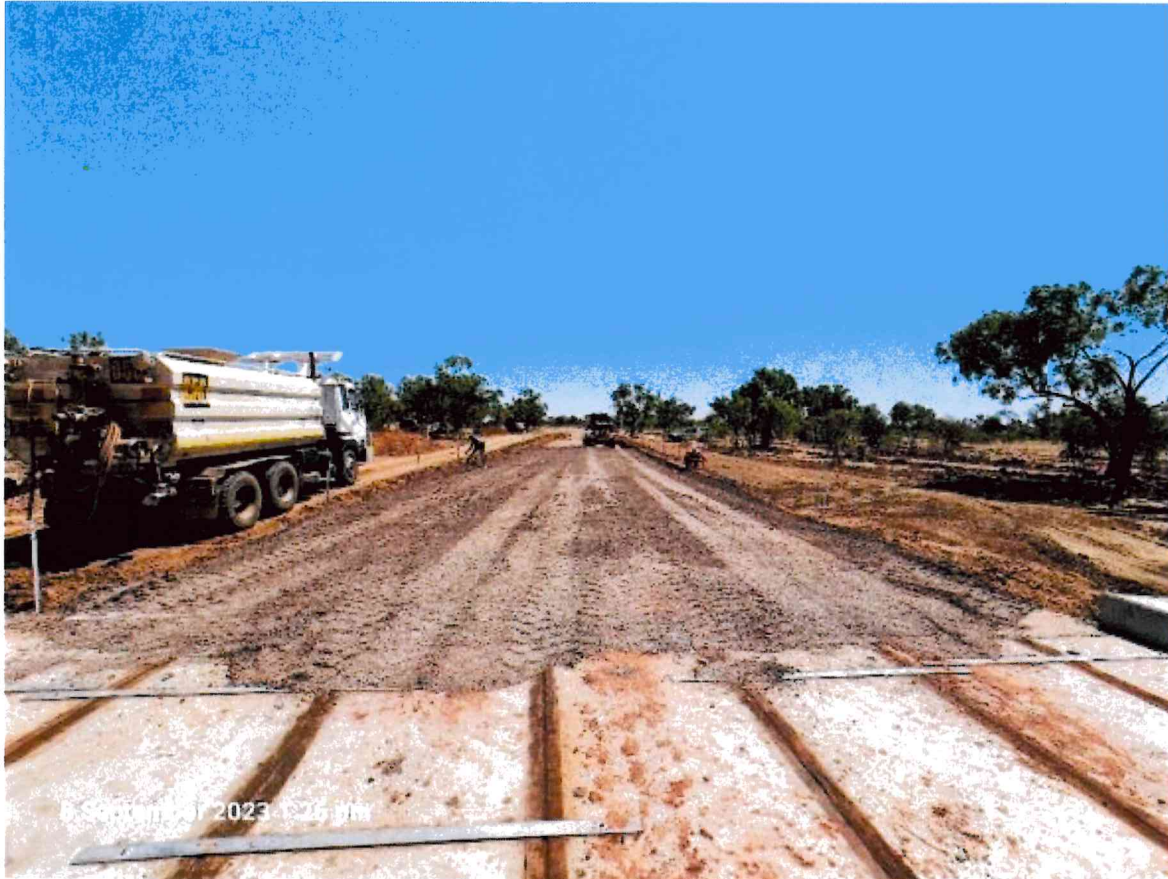
Figure 5: Doomadgee East Road Culvert, placement of road base
