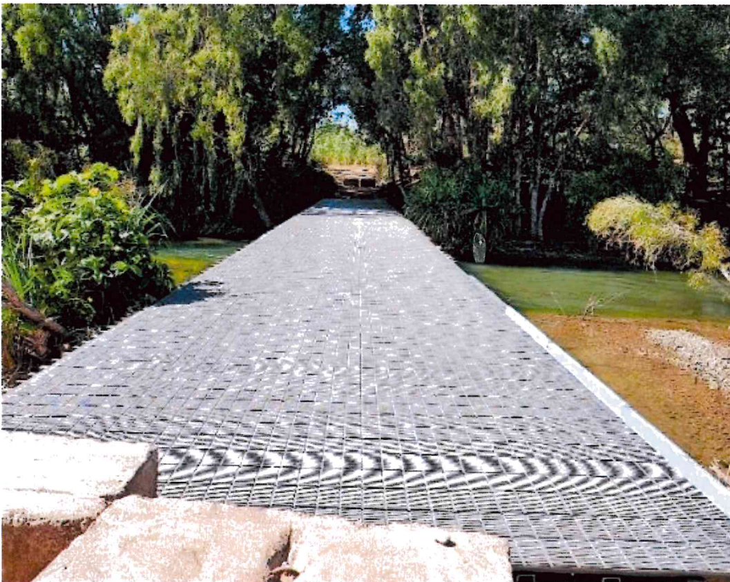
Figure 6: Completed deck and the progress of installation of bridge kerb of Gregory Service Bridge
