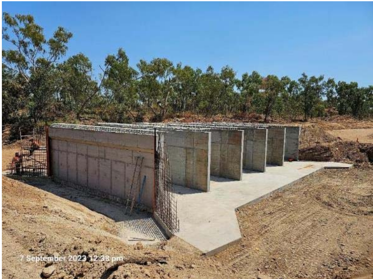
Figure 4: Archie Creek Culvert walls
