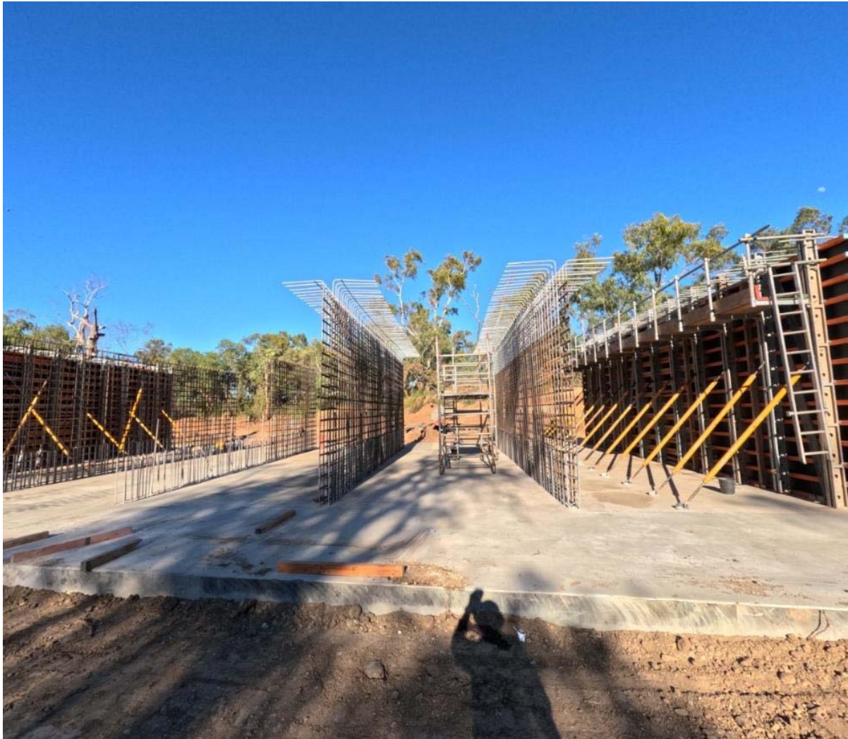
Figure 4: Archie Creek Culvert walls
