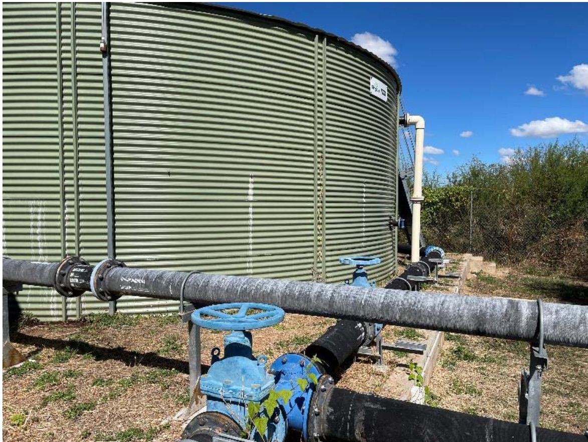
Figure 1: Gregory Water Treatment Plant, existing reticulation (due for the upgrade) and the Reservoir (will be relined)
