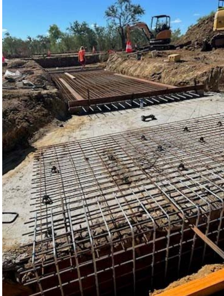
Figure 5: Doomadgee East Road Culvert, base slab reo works
