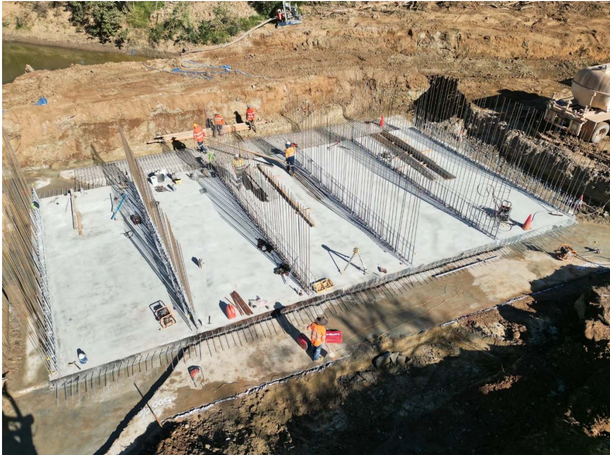
Figure 4: Archie Creek Culvert, Base slab and reinforcing
