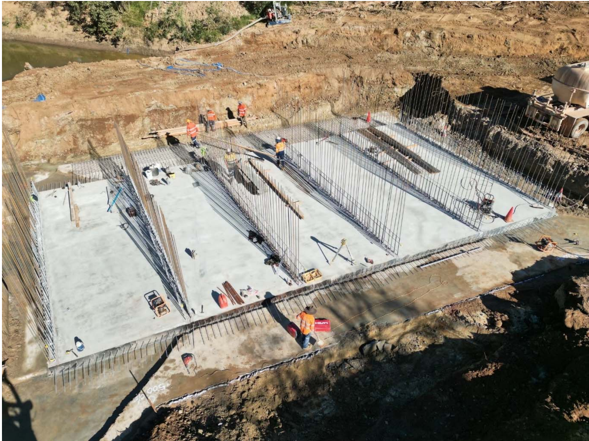
Figure 4: Archie Creek Culvert, Base slab and reinforcing
