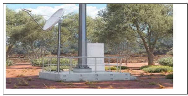
The height of the proposed structure is a 20metre monopole with various antenna increasing the overall height to 21.4 metres.
