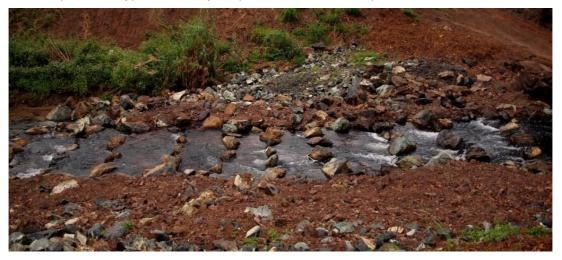
The rock ramp fish-way design also facilitates downstream fish passage, particularly by avoiding any sharp vertical drop as fish are swept downstream by flows and by providing slower flow zones which will act as refugia for fish moving downstream.
