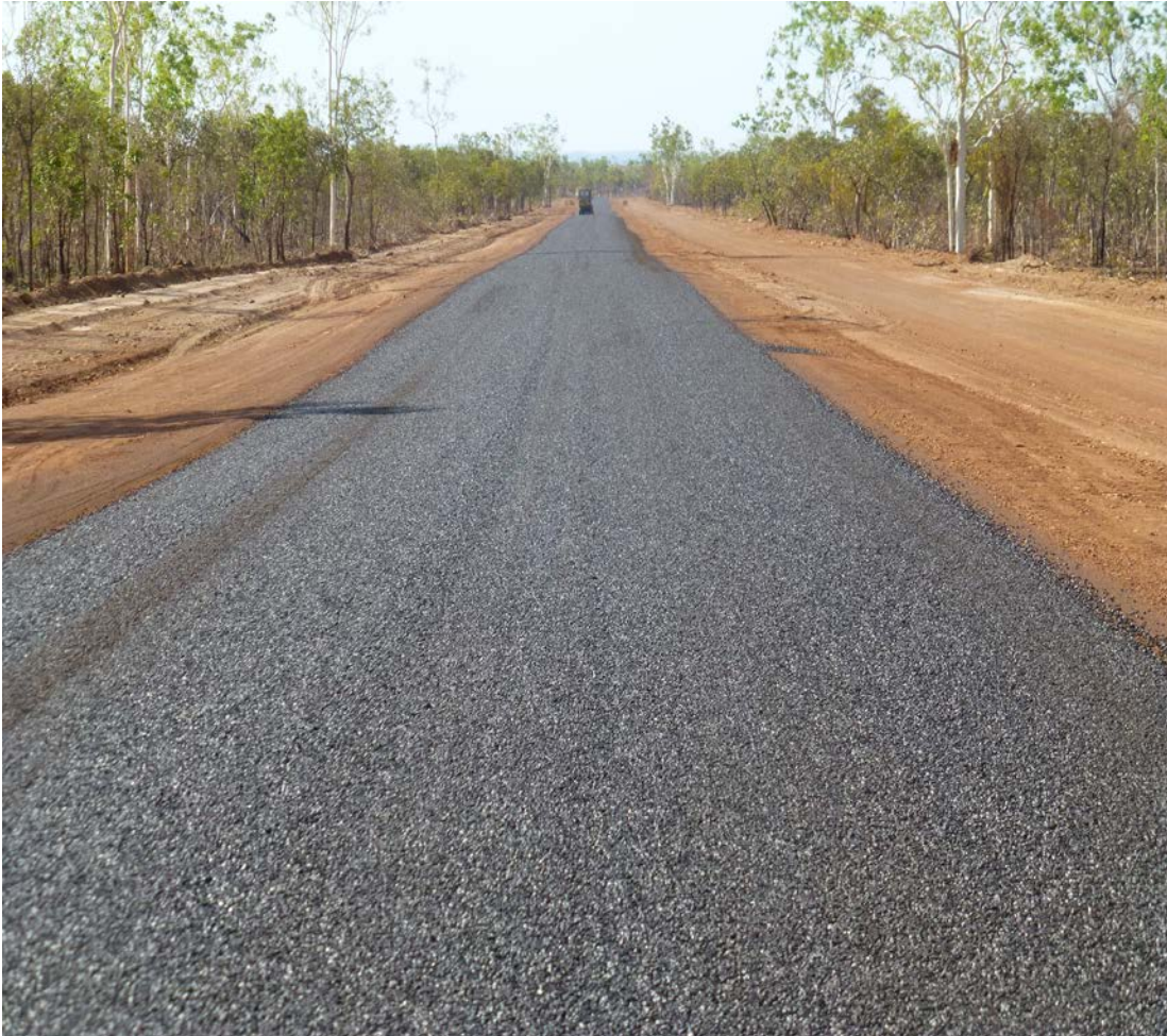
Image: sealing works on Doomadgee West Road.
