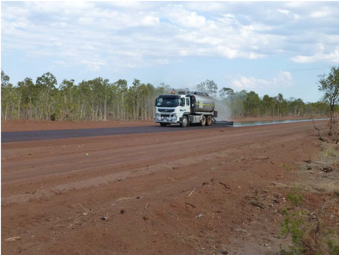
Image: Sealing work on the Doomadgee West Road.
