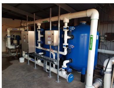
New pipes & filters for water treatment plant
