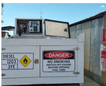
Self bunded fuel storage tank with new fuel management system
