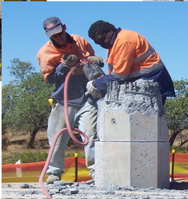
Jackhammering concrete to expose reinforcement for the next stage
