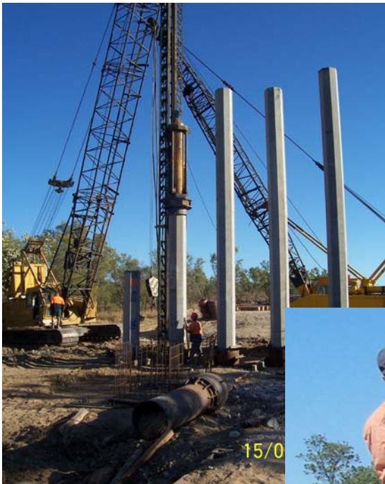
PSC piles being driven in by 4t hammer
