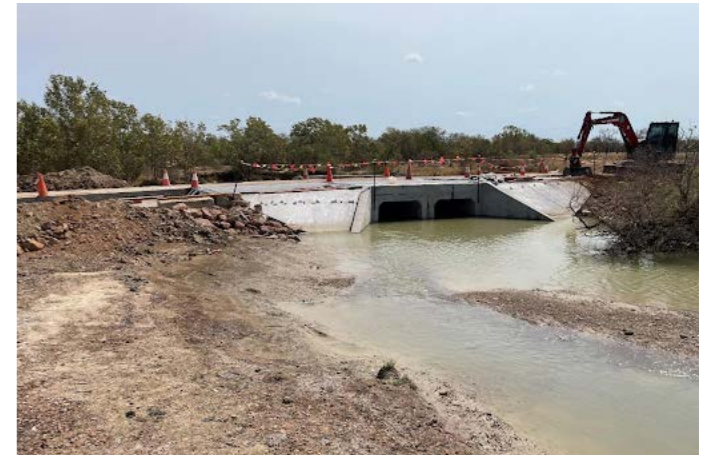
Truganini Road Beacon Pile Gully new culvert
