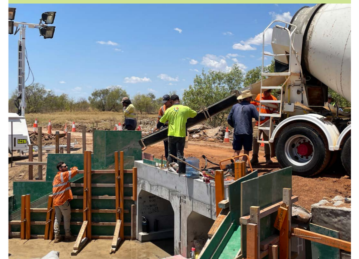
All hands on deck as they pour concrete for the new culvert
