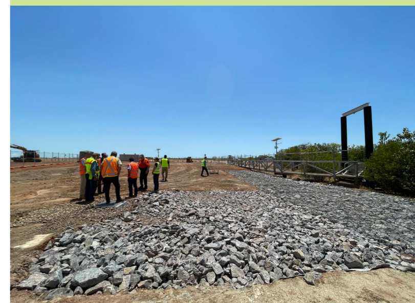
Councillors and the Burke Shire Council Engineering team inspect the new rock protection at the Wharf Recreational Grounds, which is designed to control erosion.
