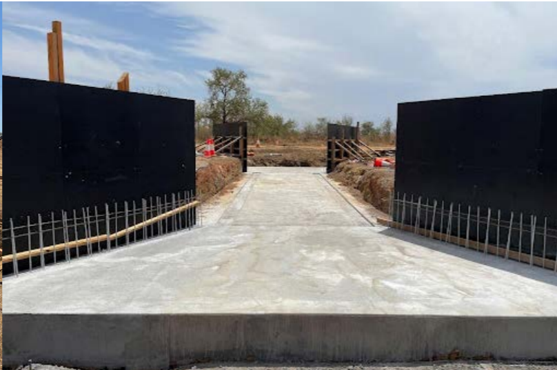
Slab of the culvert at CH 350
