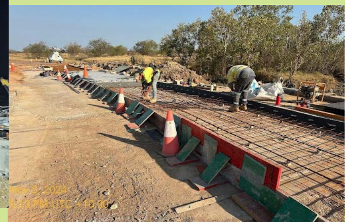
The causeway slab, being completed in two halves for traffic management reasons
