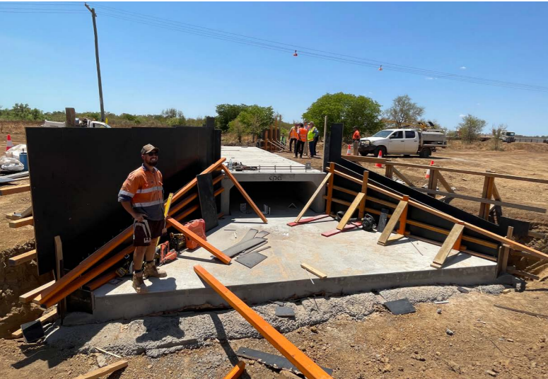
Preparing culvert for concrete pouring
