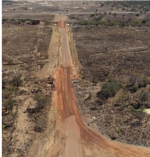
Figure 1: Burketown Airport Road alignment, de-grassing commenced
