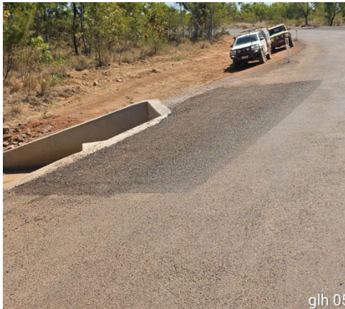
Figure 19 — Gregory–Lawn Hill Road: Patch Repairs August 2026
