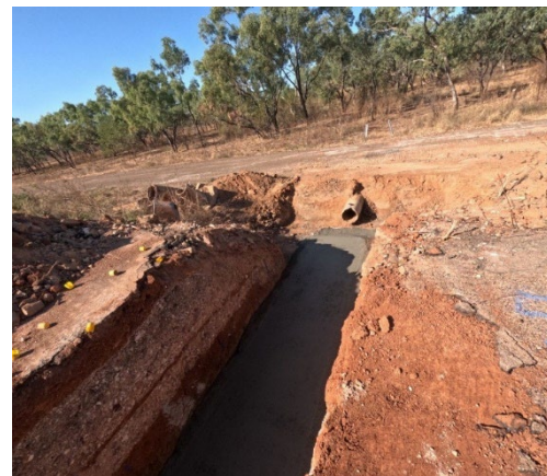
Figure 11 — Floraville Road: Stage 7 culvert base excavation, September 2026
