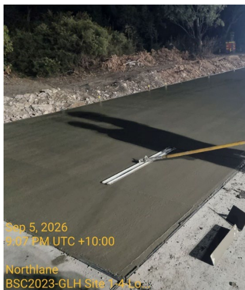
Figure 6 — Gregory–Lawn Hill Road: Road Pavement Pour, Site 4, September 2026
