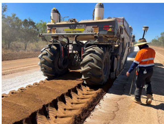
Figure 12 — Doomadgee East Road: lime stabilisation and depth verification, Zone 11, August 2026
