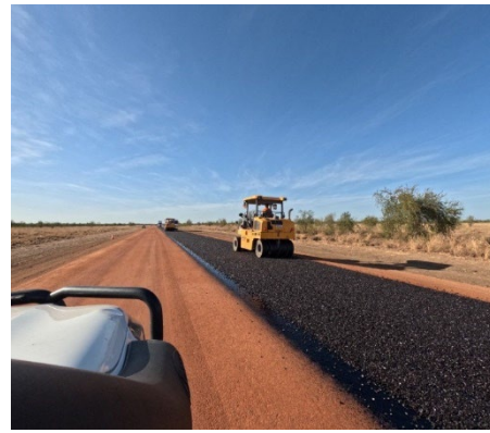
Figure 9 — Floraville Road: two-coat seal, Zones 9 and 11, August 2026
