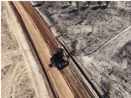
Figure 8 — Floraville Road: grading and trimming, Zone 12, September 2026
