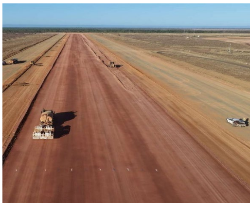
Figure 1 — Burketown Airport: MARCO rolling of the second Type 2.1 layer with third layer placement following, September 2026
