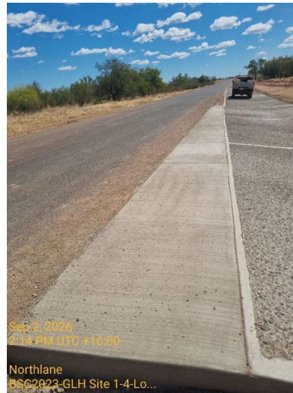
Figure 5 — Gregory–Lawn Hill Road: completed shoulder pavement, September 2026
