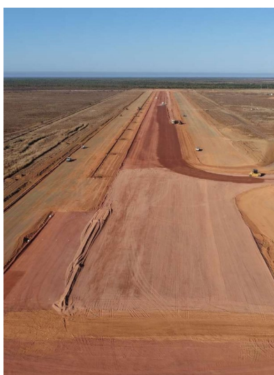
Figure 3 — Burketown Airport: Main Runway pavement looking up chainage, September 2026
