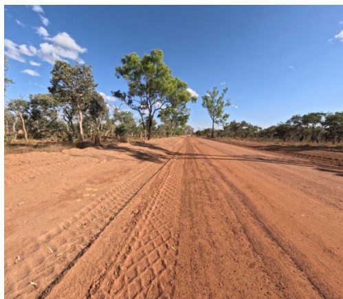
Figure 15 — Doomadgee–Lawn Hill Road: completed formation and pavement, August 2026
