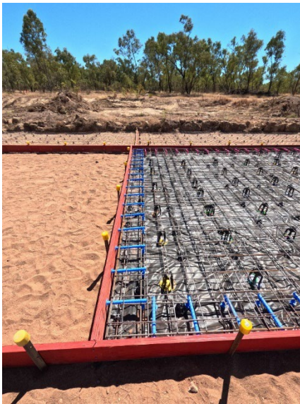
Figure 4 — Gregory–Lawn Hill Road: reinforcement and dowel placement, Site 4 concrete pavement, August 2026
