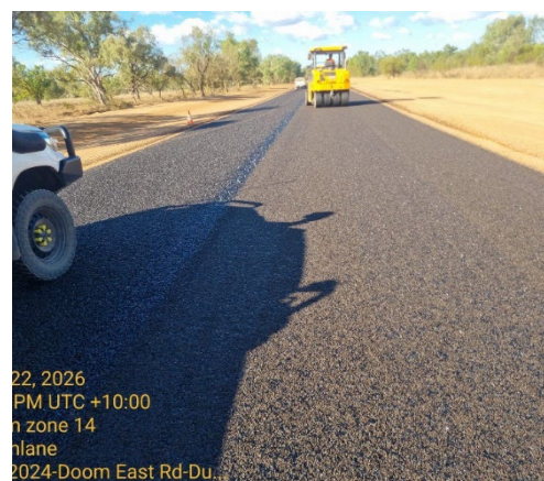
Figure 13 — Doomadgee East Road: two-coat seal complete, Zone 14, August 2026
