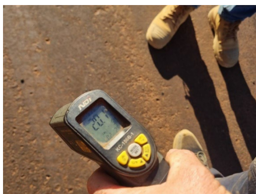
Figure 21 — Doomadgee East Road: seal spray rate and temperature verification, August 2026
