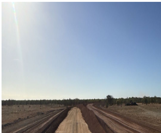
Figure 10 — Floraville Road: Type 2.1 base course import, Zone 10, September 2026
