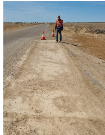
Figure 20 — Gregory–Lawn Hill Road: cement stabilised patch repair, August 2026
