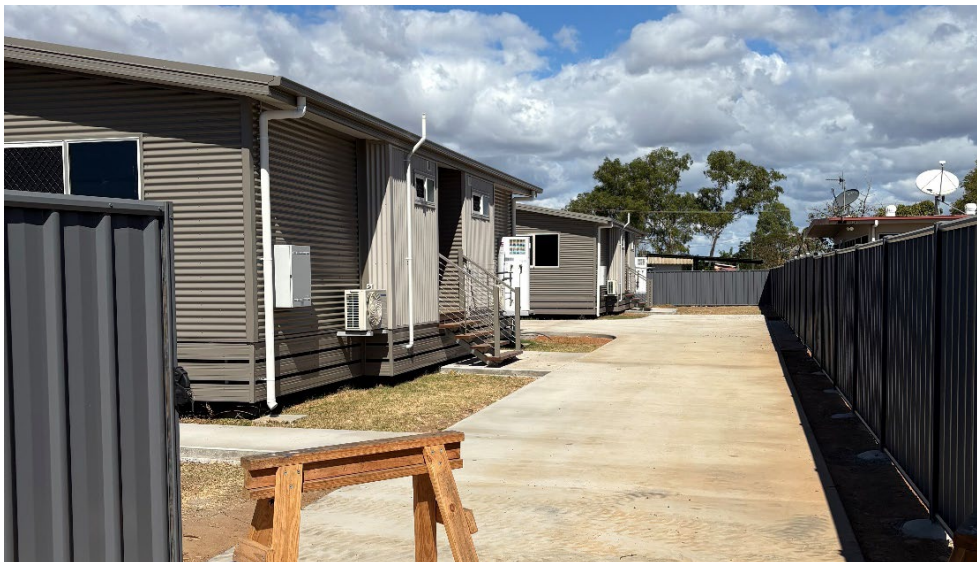
Figure 3: 41 Musgrave St units, fencing and driveway completed.
