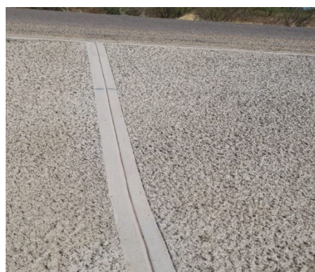
Figure 22 — Gregory–Lawn Hill Road: concrete pavement joint inspection, Site 4, September 2026
