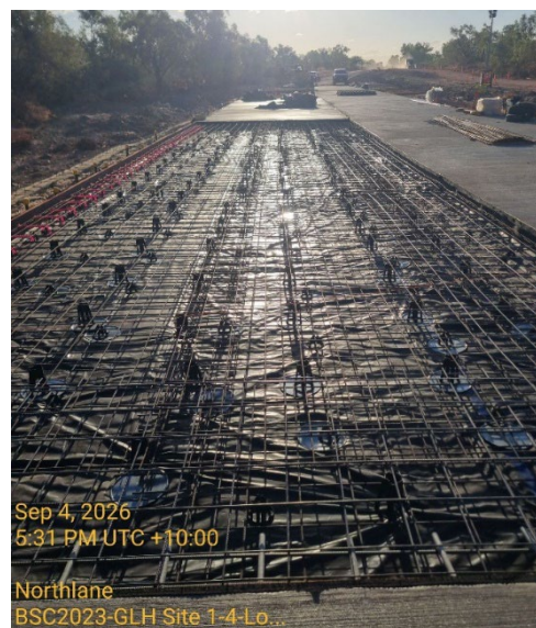
Figure 7 — Gregory–Lawn Hill Road: Road Pavement Pre-pour inspection, Site 4, September 2026
