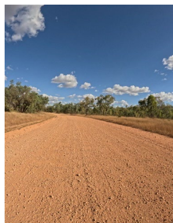
Figure 18 —Lawn Hill National Park Road: Completed grading works – August 2026
