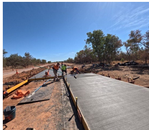
Figure 10 — Floraville Road: new concrete floodway at ch 9080, August 2026
