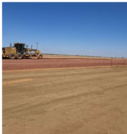
Figure 4 — Trimming and grading of the Main Runway pavement, August 2026
