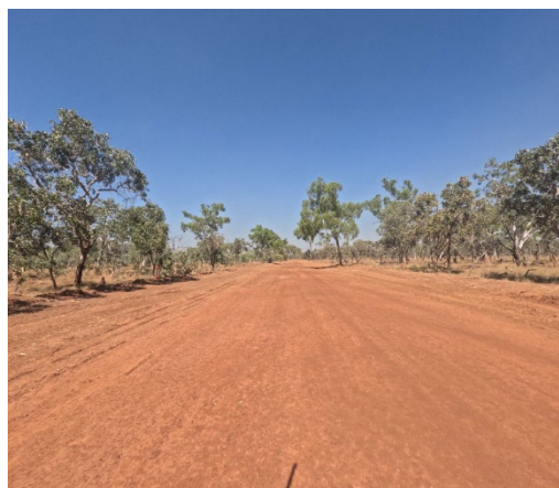
Figure 13 — Works complete – Doomadgee Lawn Hill Road
