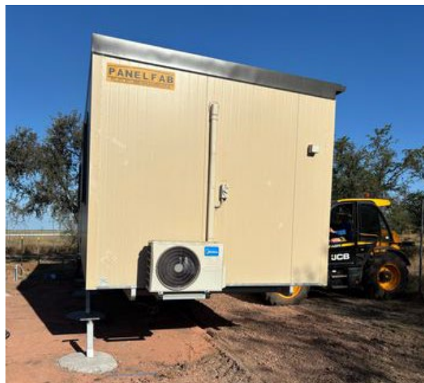
Figure 2: Gregory SES donga during the installation
