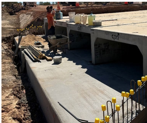
Figure 9 — Floraville Road: Stage 5 Culvert 1 box culvert installation, August 2026
