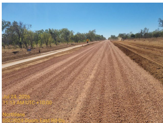
Figure 11 — Doomadgee East Road: pavement placement, Zone 16, July 2026
