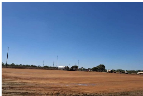
Figure 2 — Completed apron lower sub-base stabilised layer, August 2026
