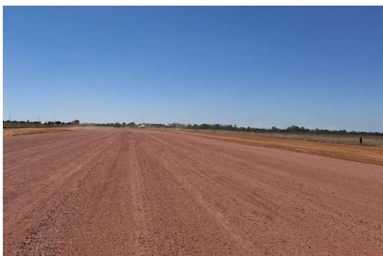
Figure 1 — Type 2.1 base course placement on the Main Runway, August 2026
