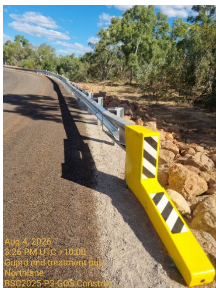
Figure 15 — Gregory–Lawn Hill Road: guardrail and end treatments complete at Archie Creek, August 2026
