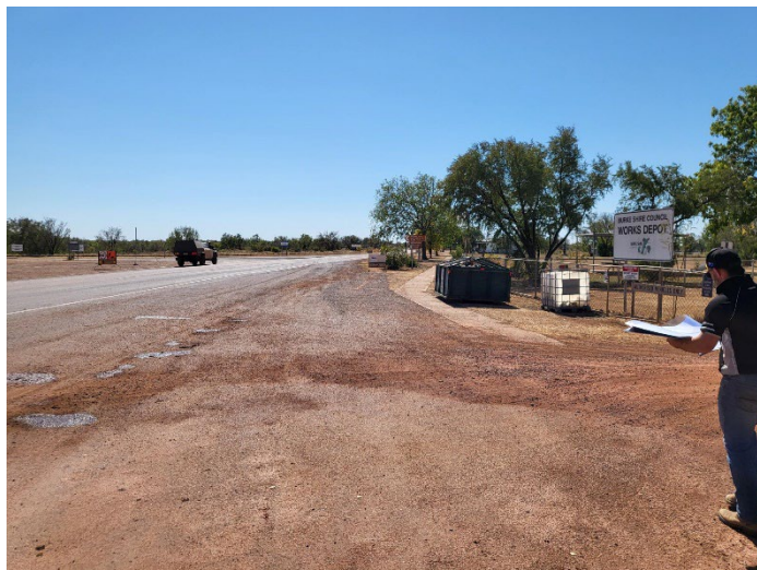
Figure 3: Gregory Stormwater Contract (Stage 1 of Gregory Town Street Reconstruction) kick off meeting, proposed alignment
