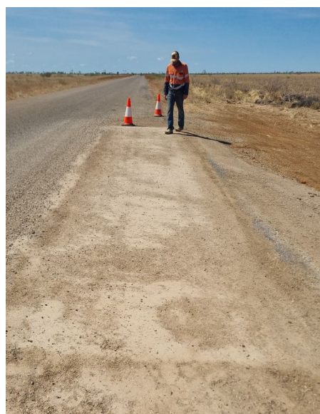
Figure 16 — Gregory–Lawn Hill Road: cement stabilised patch repair, August 2026
