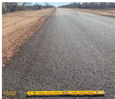
Figure 18 — Patch repair inspection, July 2026
