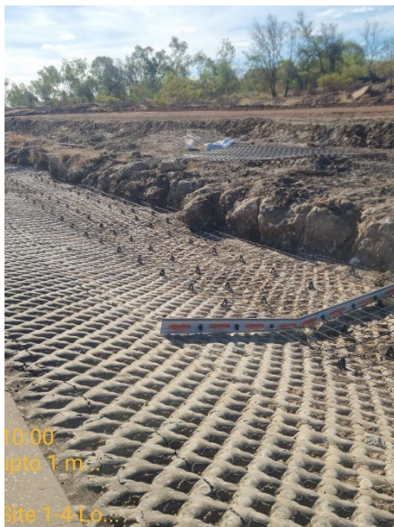
Figure 5 — Site 4: preparation of existing mattresses, August 2026
