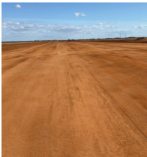
Figure 3 — Main Runway with Type 2.5 sub-base placement complete, August 2026
