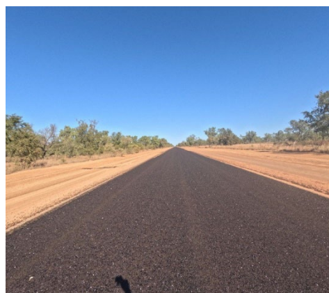
Figure 12 — Doomadgee East Road: seal complete, July 2026
